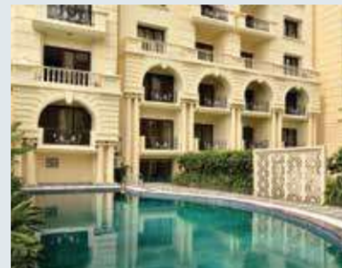
SHALIMAR EMERALD JOPLING ROAD
