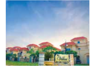
SHALIMAR PARADISE LUCKNOW - FAIZABAD ROAD UPRERAPRJ9777
