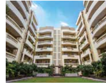
SHALIMAR DWELLING AP SEN ROAD LUCKNOW
