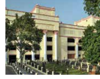
MULTILEVEL PARKING HAZRATGANJ LUCKNOW
