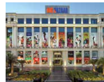
SHALIMAR ELLDEE PLAZA BHOOTNATH MARKET LUCKNOW
