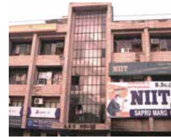
SAS HOUSE SAPRU MARG LUCKNOW
