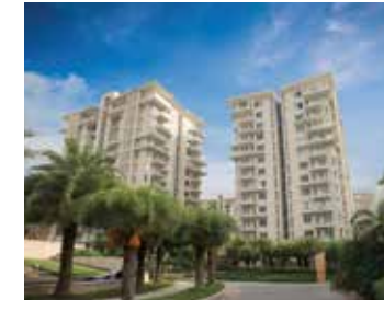
SHALIMAR GALLANT MAHANAGAR LUCKNOW UPRERAPRJ3168
