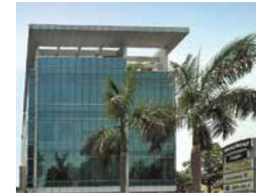
SHALIMAR LOGIX RANA PRATAP MARG LUCKNOW
