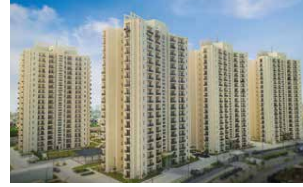
VISTA GOMTI NAGAR EXTENSION LUCKNOW - UPRERAPRJ4833
