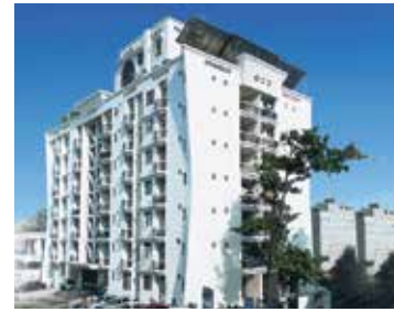
SHALIMAR APARTMENTS P. N ROAD LUCKNOW
