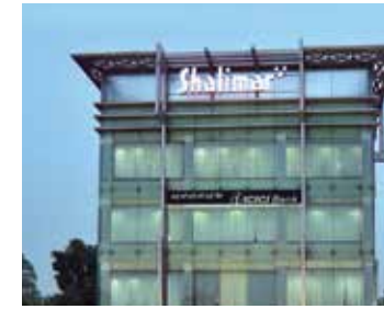
SHALIMAR STAR, HAZRATGANJ, LUCKNOW
