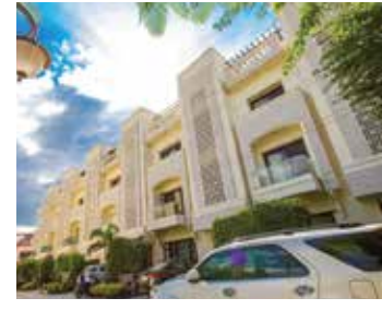
SHALIMAR MEADOWS GOKHALE MARG LUCKNOW
